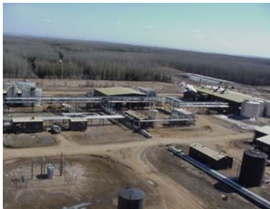
Dover SAGD Facility
