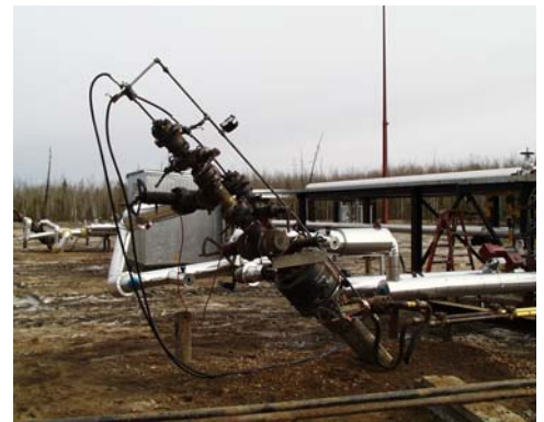
Dover Vapex Pilot Project
